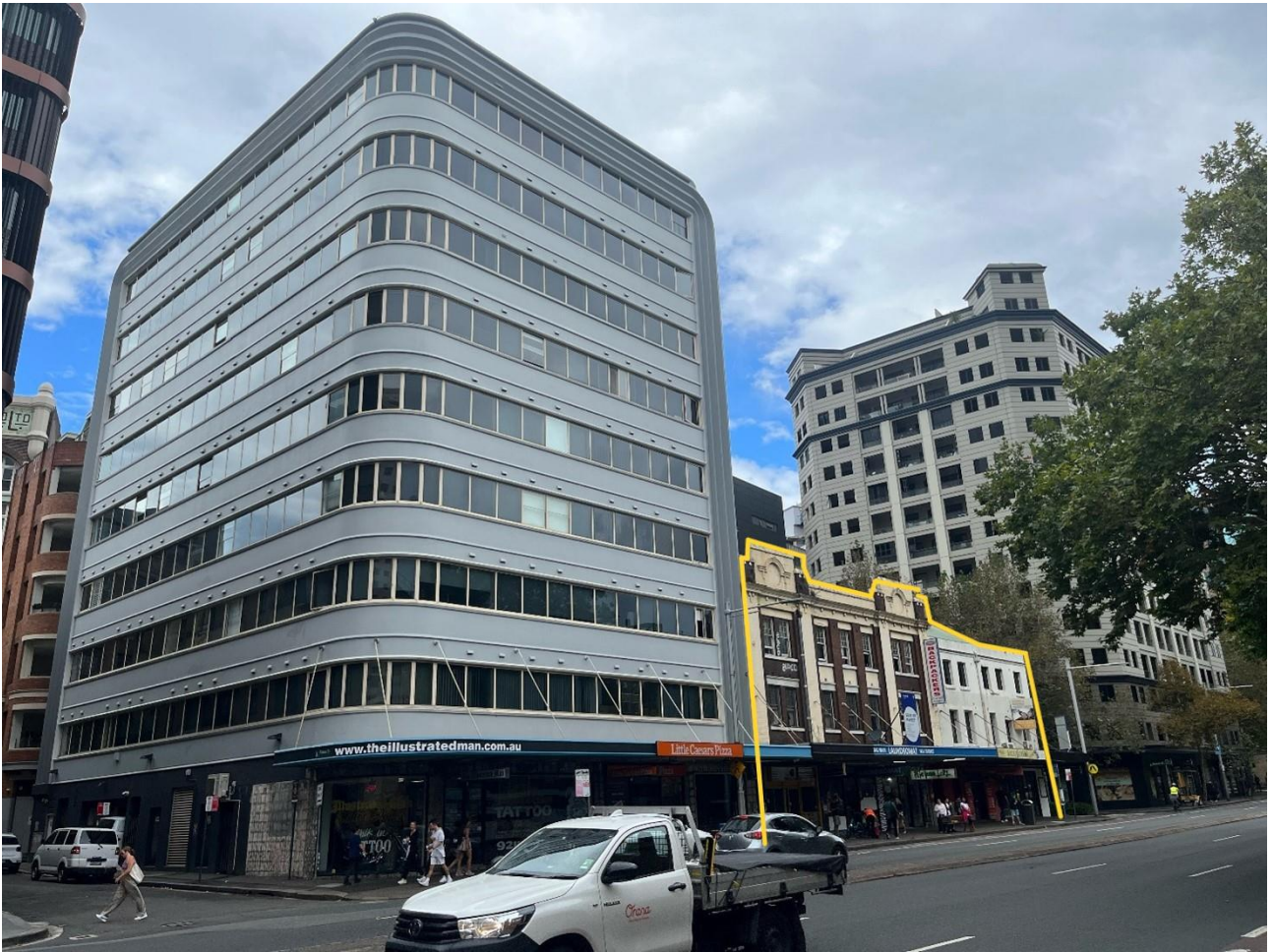
Figure 4. 232-240 Elizabeth Street, viewed from the north-west, outlined in yellow
